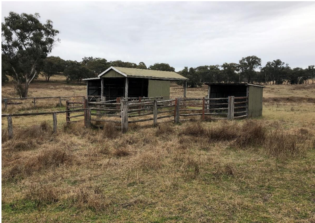
Figure 2.3: Photo A –Existing sheep/cattle yards (Lot94//DP755426) in a north-west direction
